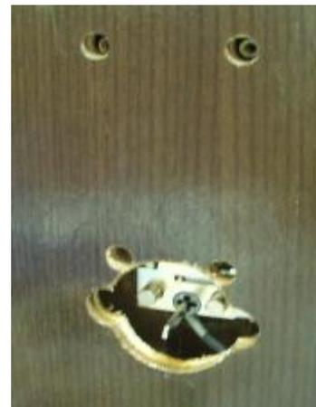
2、 Attach the exterior part of the lock on the door. (Press the lock against the door, and check the length of the torque bar is the same as the thickness of the door (The standard of the torque bar: the lengthen of the torque bar is the same as the door thickness or 0-3mm less is also acceptable.)
