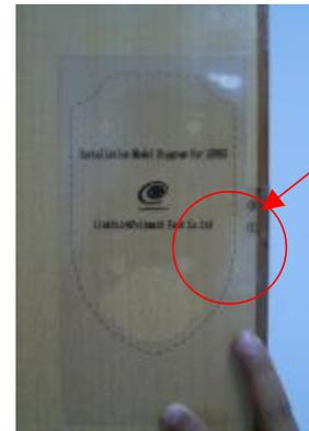
Tape the template onto the door to mark down the hole position.
