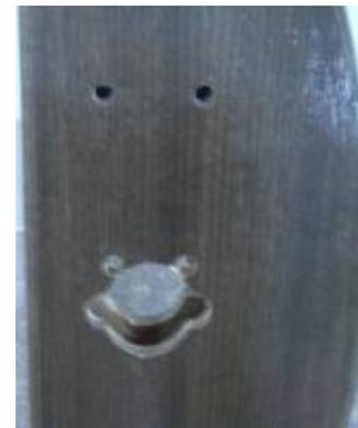
3.Insert the latch through the latch bolt hole on the edge of the door. Secure the latch into the door with the screws provided with the lockset. Keep the "UP" mark on the latch always upside.
